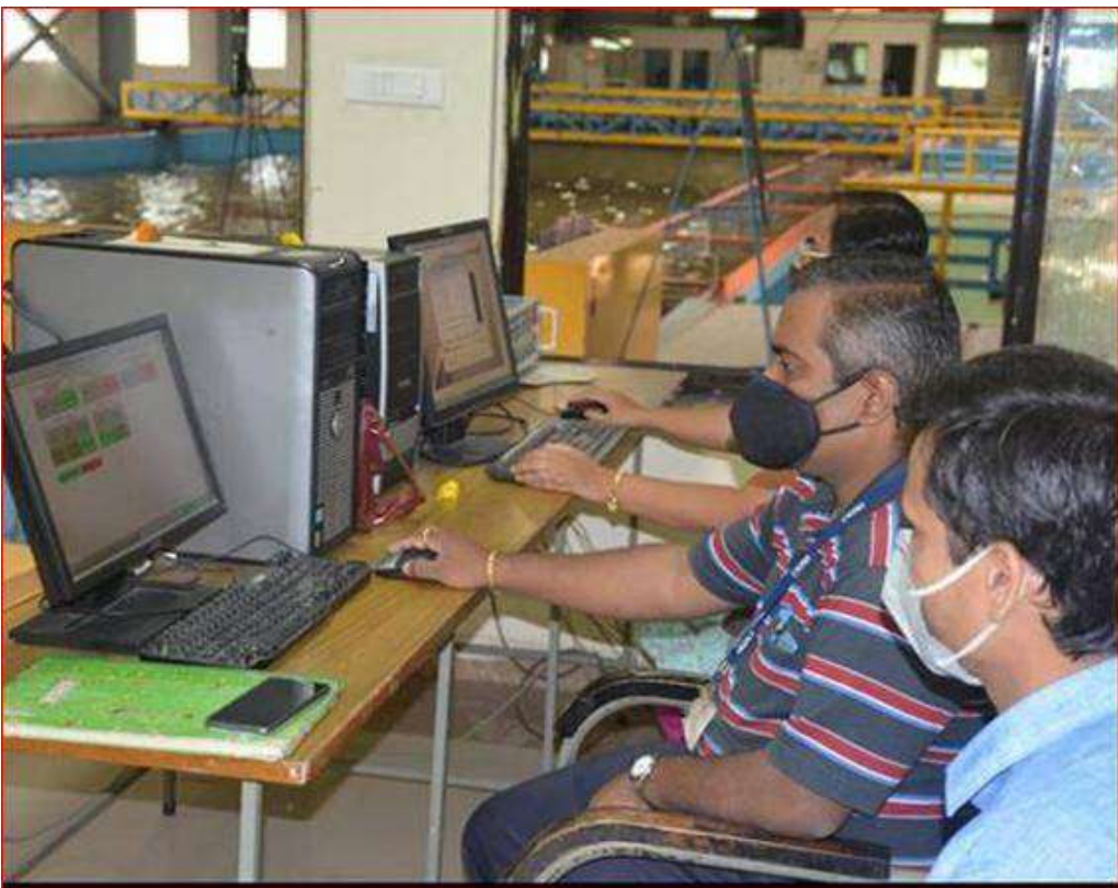
Photo-4 : Control room with wave data acquisition System
